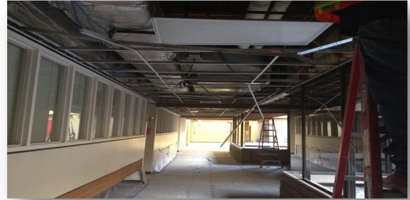
TPHS – B Building
